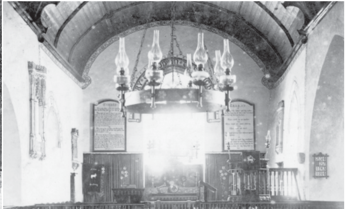
The inside of the St. John's Church in the 1920's.
