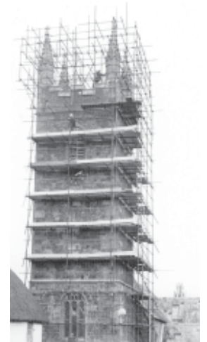
In the 1960's repair work was carried out on the Church tower.
